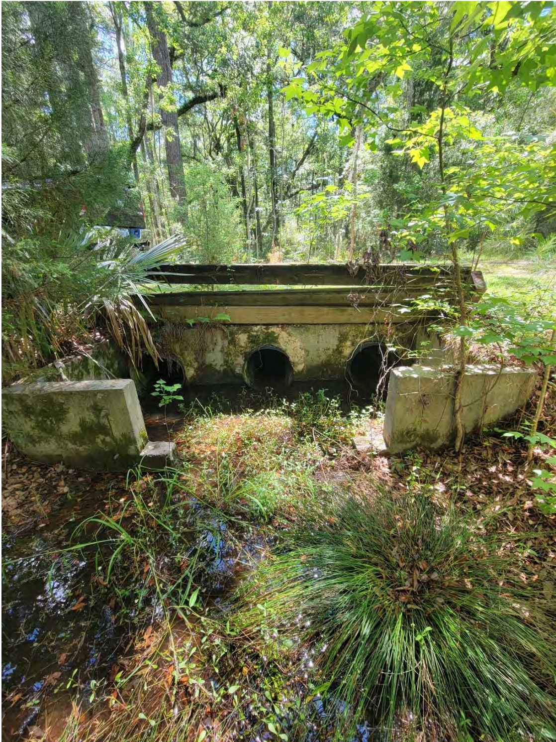
Figure 7. View of the cement structure attached to some drainage pipes in the Bird Sanctuary which may be the remnants of a flashboard riser water control system.
